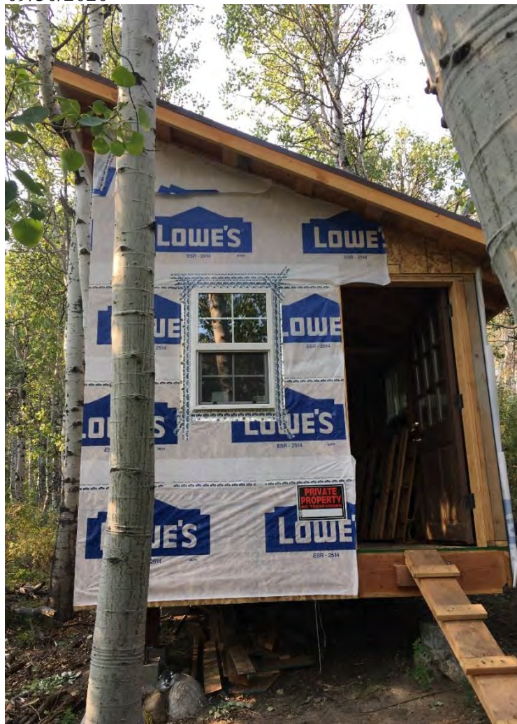
Existing 116-square foot shed, looking west.
