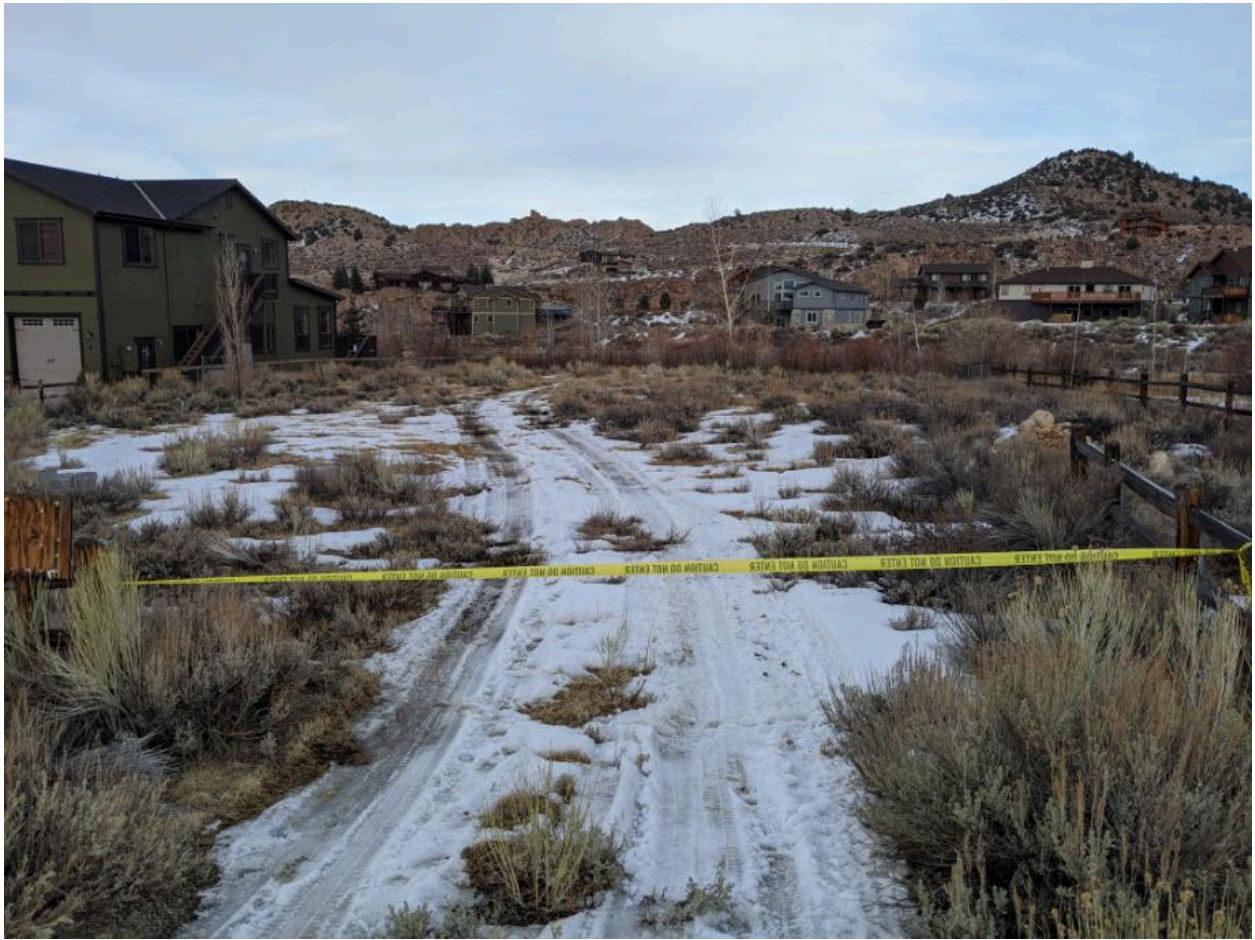
The manhole is located at the far corner of this lot. Caution tape has been placed to prevent access to the lot.
