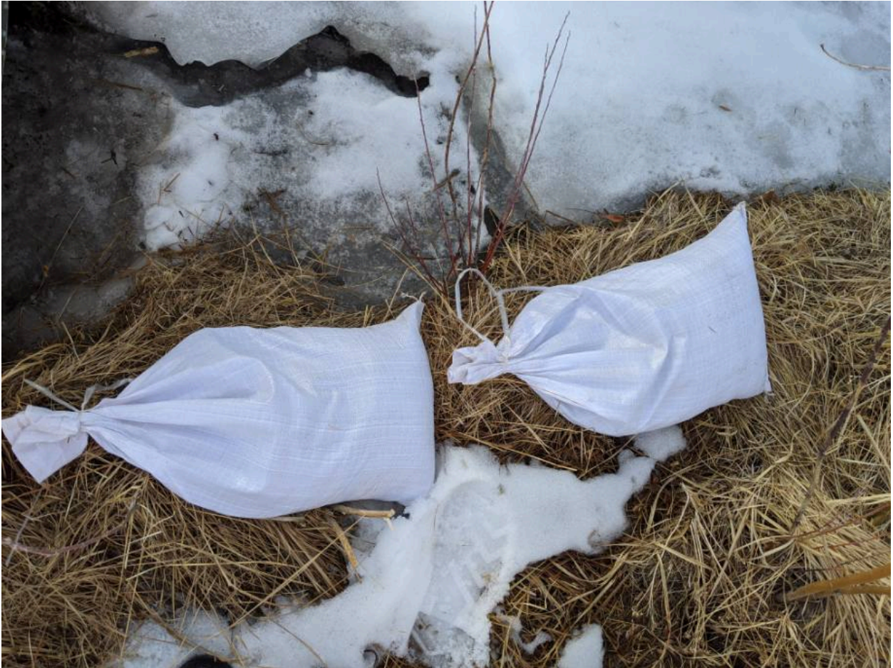
Sandbags placed in two low points for snow-melt runoff
