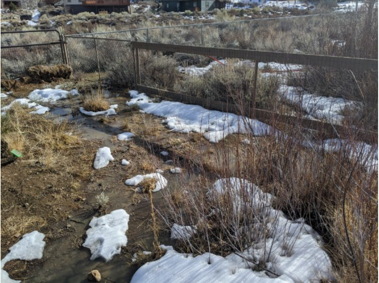
Area of flow from the backyard of 74 Sierra Springs Drive
